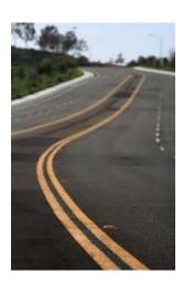
Signing and striping are used to help reduce speeds in residential areas. Striping creates narrow lanes that give the illusion of a narrow street. Signing enforces speed reduction with the use of speed limit signs and/or neighborhood signs.
